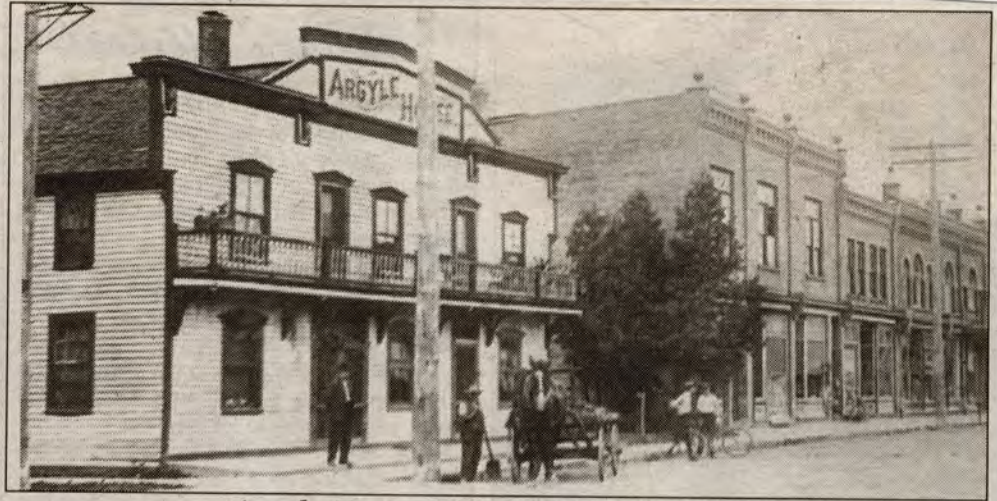
Argyle House 1870s-1961, West Lorne
